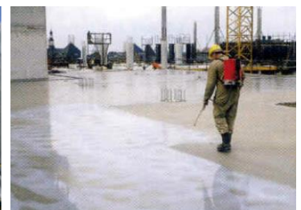
Aanbrengen curing compound
